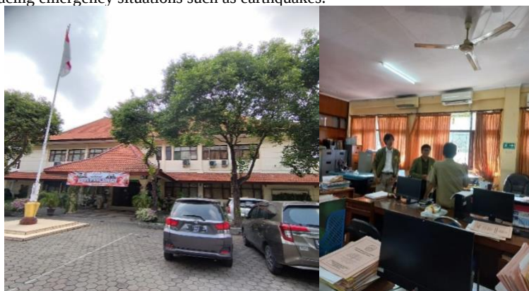
Figure 3: Direct observation of the East Java Provincial Environmental Service Building and interviews with employees of the East Java Provincial Environmental Service Building
