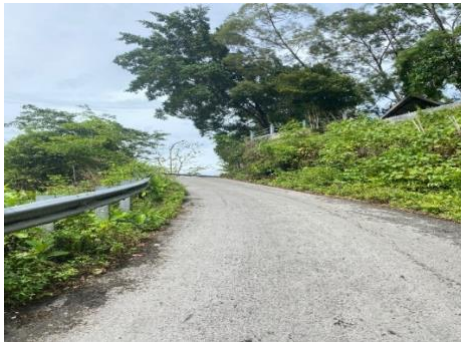
Figure 3 (b). The road is not equipped with signs, markings, and street lighting
